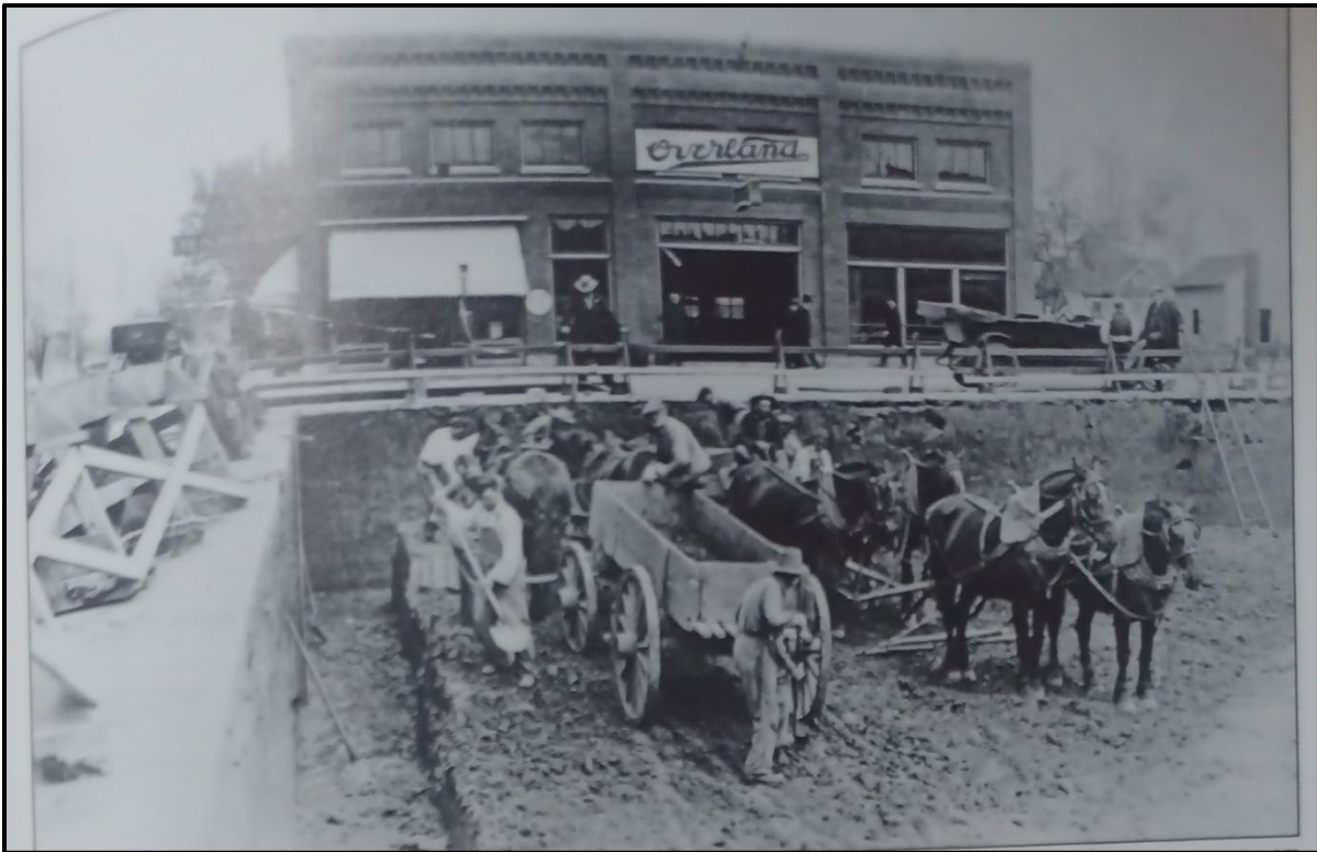
Figure 14. A 1904 photo of a crew digging out a basement for the Taylor-Dale Hardware Building (608 3 rd St.). The O'Dell Building is visible in the background, being used by the Overland Automobile Co. (Van Heukelem and Fuller 2012).
